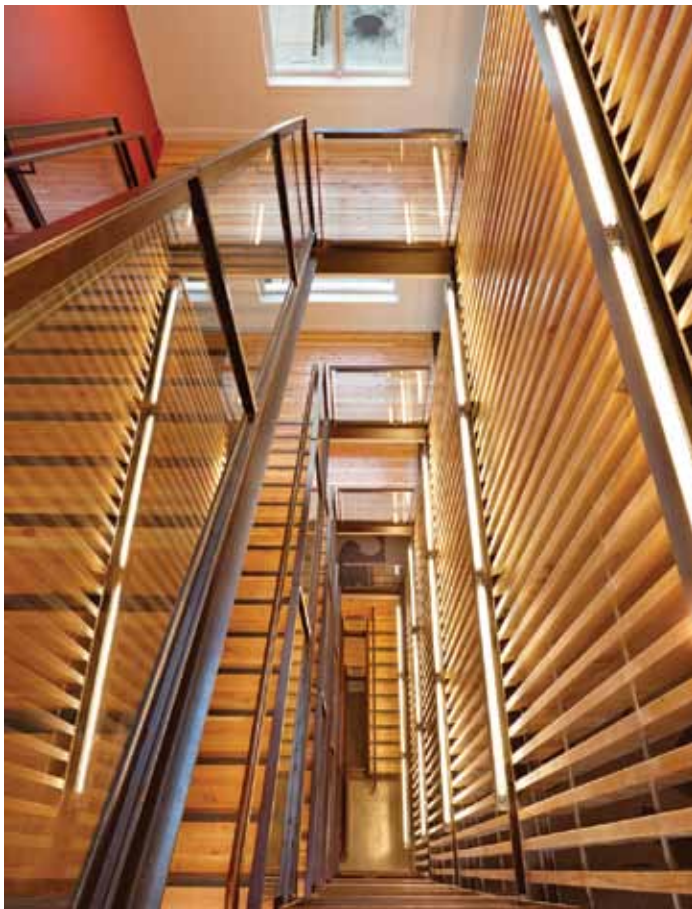
Wood was used as both a structural and finish material throughout the UW project.
