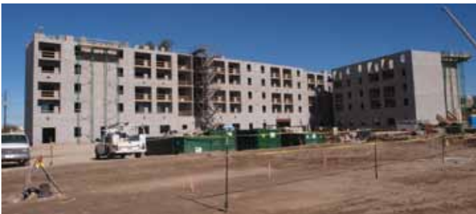
Figure 5. Building under construction.
