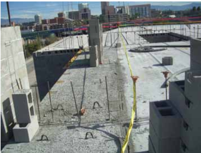
Figure 4. Plank floor with CMU bearing walls.
