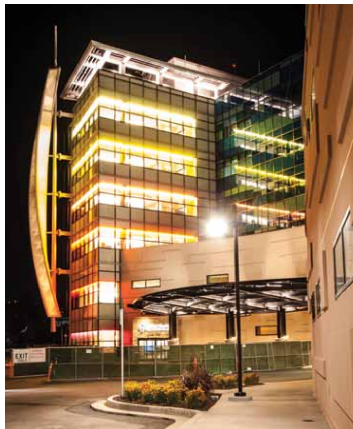
Figure 2: Sutter Health Eden Medical Center (SHEMC) Project. Courtesy of Sutter Health, Devenney Group, Christopher Skow Photography.
