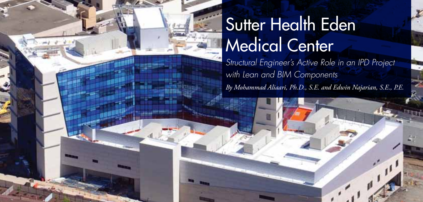
Figure 1: Sutter Health Eden Medical Center (SHEMC) Project. Courtesy of Sutter Health, DPR Construction.
