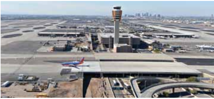
A Southwest Airlines 737 crosses over the newly completed Taxiway "S" bridge. Courtesy of Visions in Photography.
