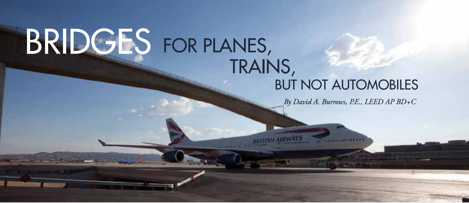
British Airways 747 crossing beneath the Taxiway "R" bridge, June, 2012. Courtesy of City of Phoenix Aviation Department.
