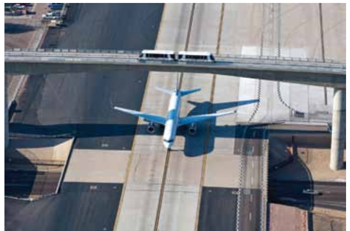
A US Airways jet passes beneath the Taxiway R crossing with the PHX Sky Train overhead. Courtesy of City of Phoenix Aviation Department.
