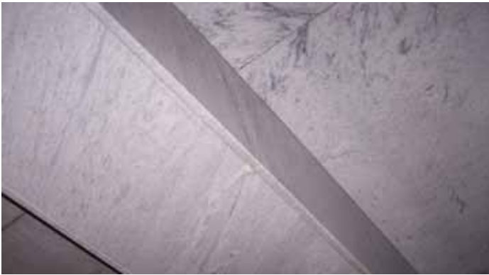
Figure 4. Typical 18- x 18-inch concrete beam enclosure in hallway.
