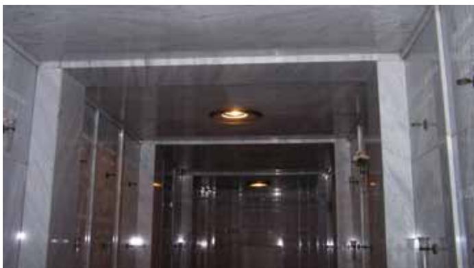
Figure 2. Interior of marble clad ceiling, beams, and walls.
