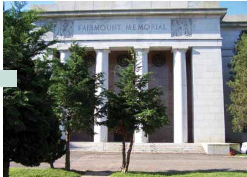
Figure 1. Exterior of the Fairmount Mausoleum.
