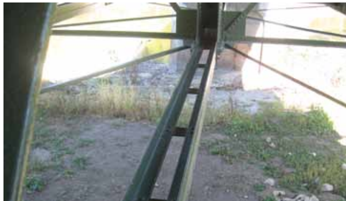
Shop-fabricated bottom chord truss member with rivets.
