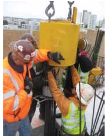
Figure 7: Hydraulic stressing jack being placed over the vertical post-tensioning tendons.
