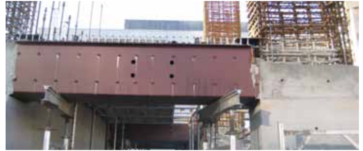
Figure 10: Link beam steel jacket.
