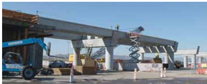
The elevated guideway under construction, showing erection of the U-beams.
