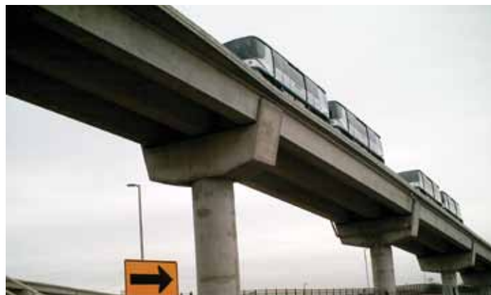
The completed elevated guideway in service.
