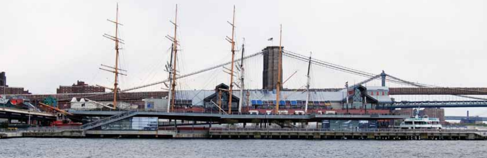
Figure 5: East River Pier 15 deck had to be raised to the flood elevation to accommodate the small pavilions below the code requirement of the FEMA flood elevation. Courtesy of Arup.
