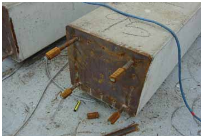
Figure 2: Plate at the bottom of the concrete which connects to the steel section. The connections use a simple detail to facilitate construction in the field. Courtesy of Hudson River Park Trust.
