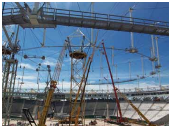
Figure 5: Temporary erection tower.
