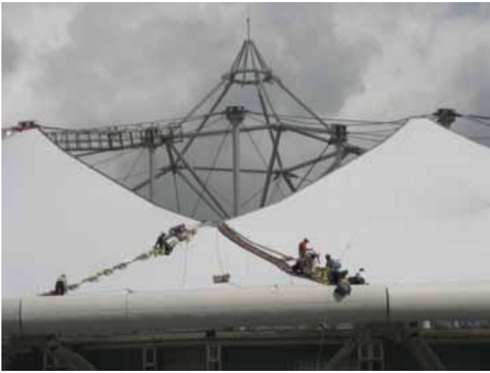
Figure 6: Installation of fabric cover over cable network.
