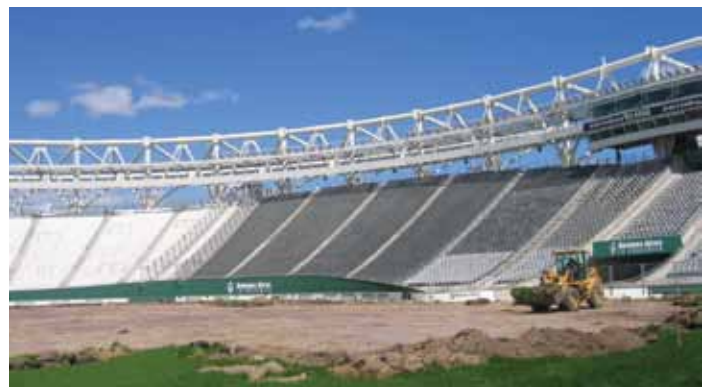
Figure 2: Interior view of compression ring.
