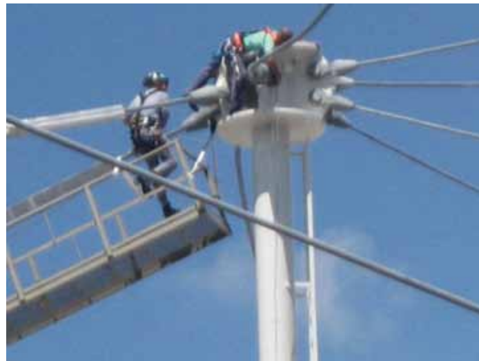
Figure 4: Attachment of cables to post.
