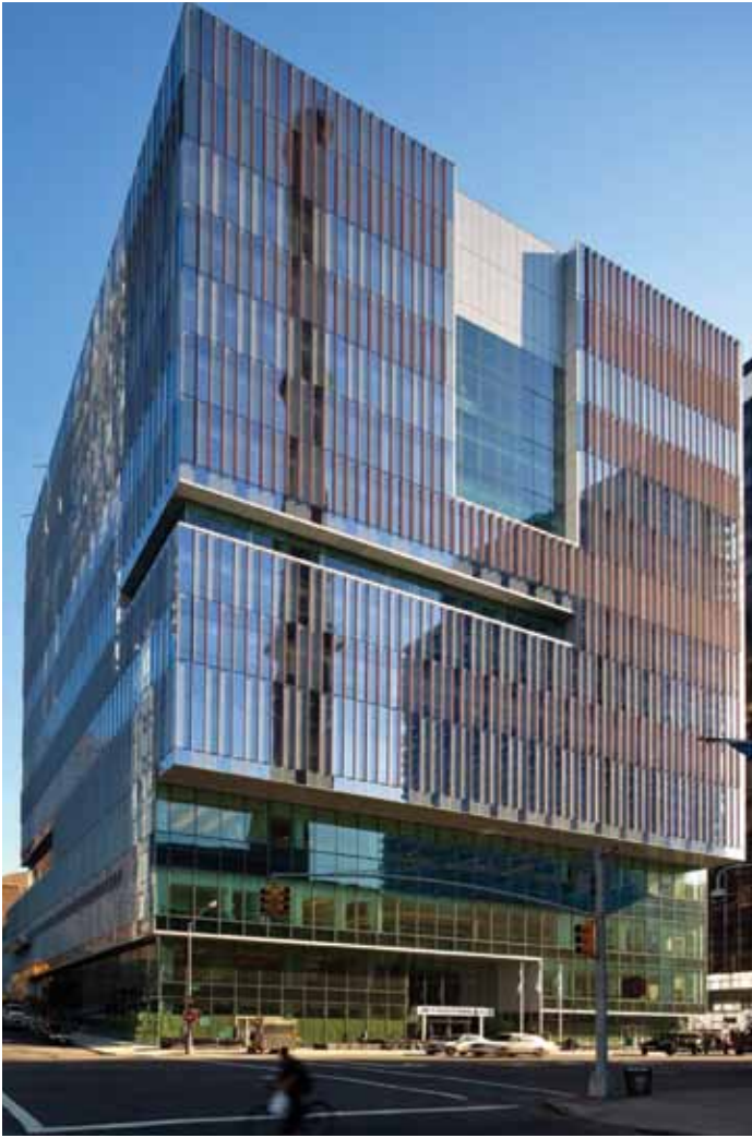
Main entrance on 11 th Avenue. Setbacks in the façade were an important aesthetic feature that also reduced the impact of the load on the shallow train tunnel below.
