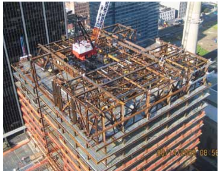
Truss construction supports the 26 perimeter hangers.
