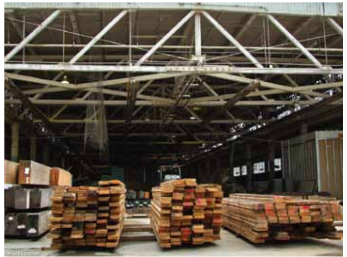
Deconstruction of the warehouse. Courtesy of Charles Lozner.
