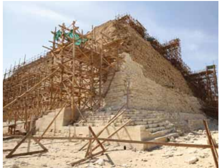
Figure 6. Scaffolding in use on the Step Pyramid.
