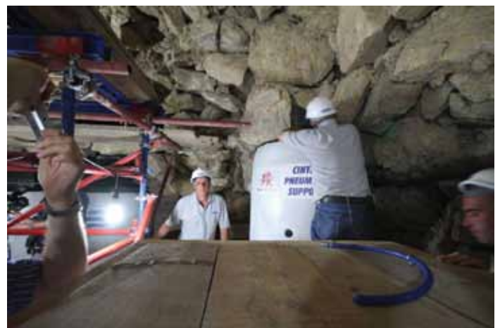
Figure 2. Cintec Waterwall airbags supporting ceiling of Step Pyramid.
