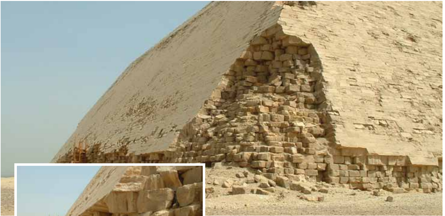
Figure 3: Major cladding damage at one corner of the Bent Pyramid.
