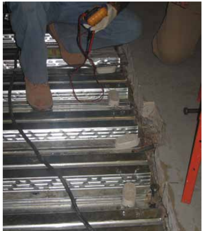
Installation of Internal Sacrificial Anode.
