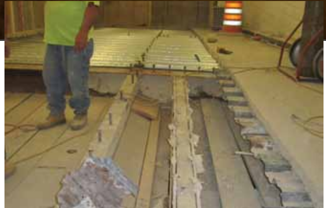
Ramp Renovation in Progress.
