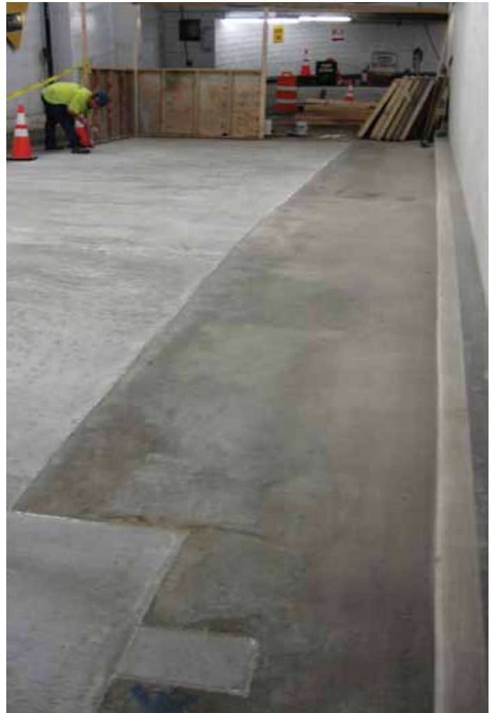
Completed Surface Repair.
