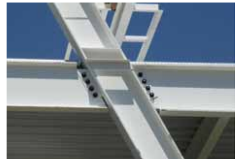
Typical bolted connection.
