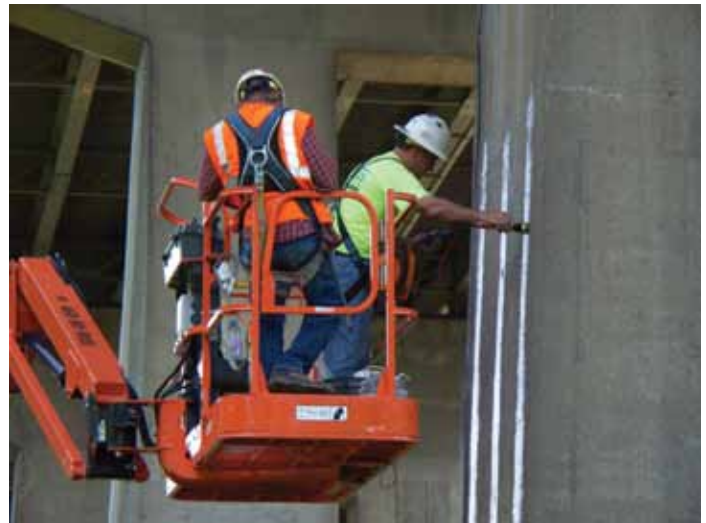
Figure 3: Measuring corrosion potential.
