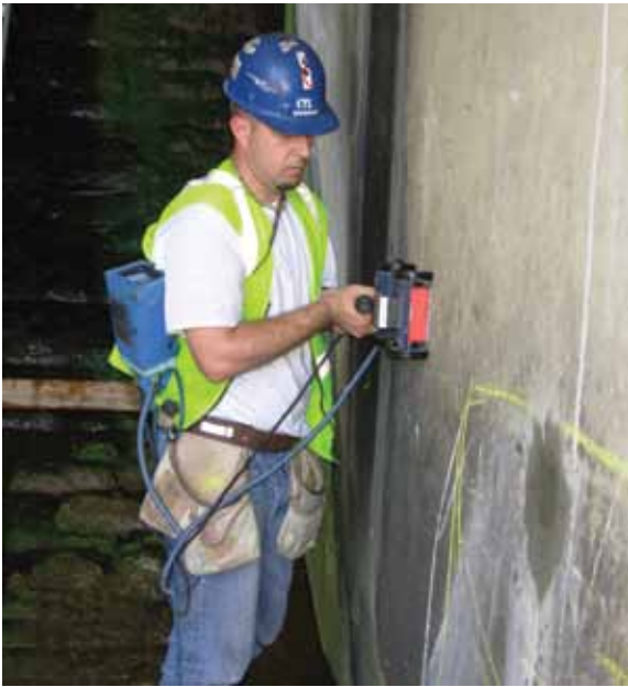
Figure 4: Collecting concrete cover profile data.
