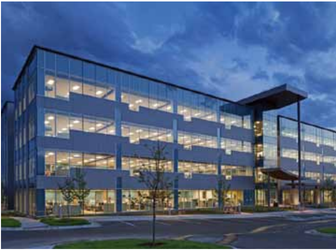
Trimble Rockies Campus completed April 2013.
