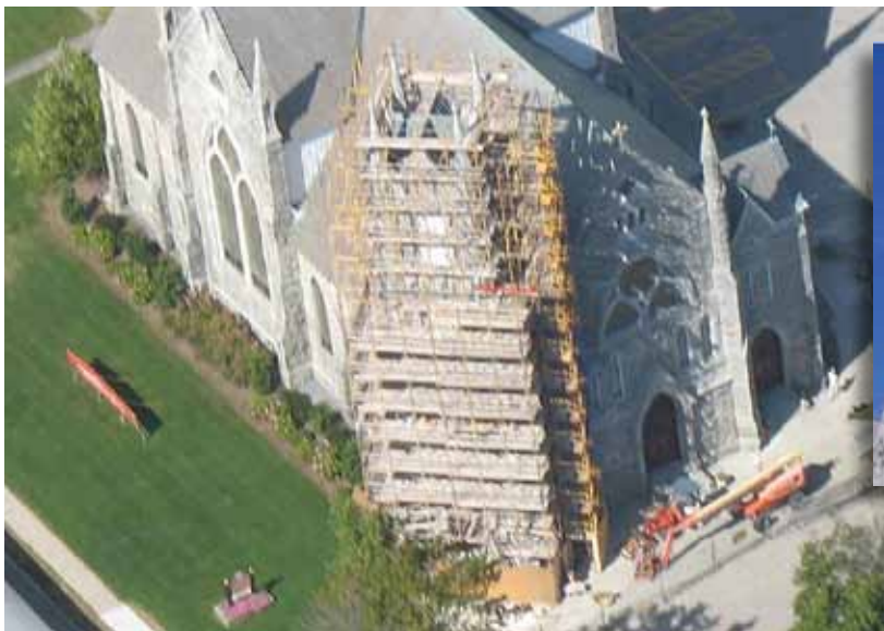
Figure 3: Tower with personnel-access scaffolding. Courtesy of Micahel Gnazzo.
