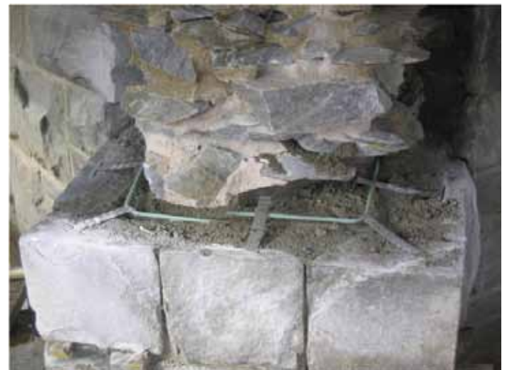
Figure 11: Stainless steel anchors to bond face stones.
