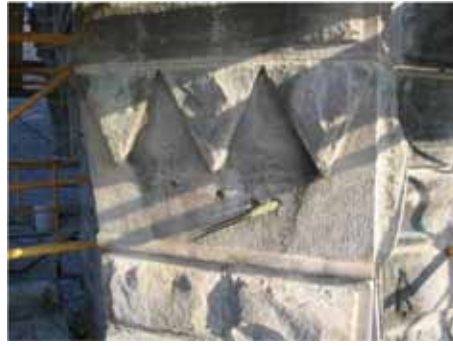
Figure 9a: Pinning upper stones before lower buttress removal.
