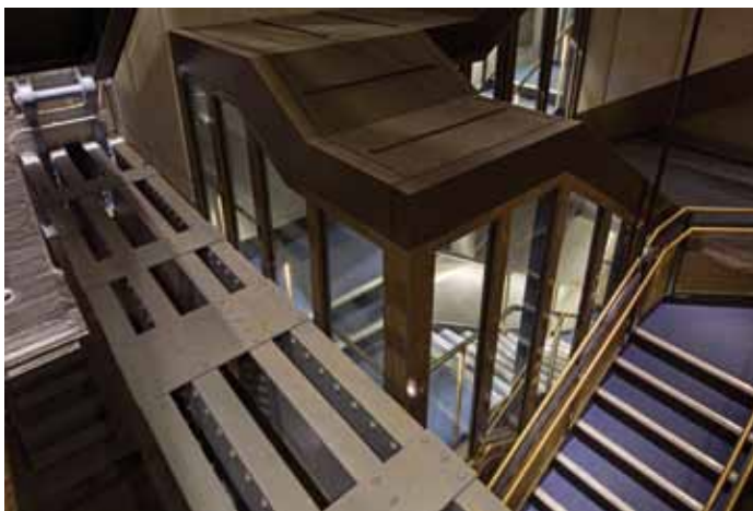
Enclosed stair structure passing through Eiffel girders between levels 3P and 4P. Courtesy of Brian Rose.
