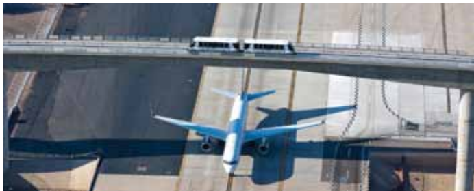
A US Airways jet passes beneath the Taxiway R Crossing with the PHX Sky Train overhead. Courtesy of City of Phoenix Aviation Department.
