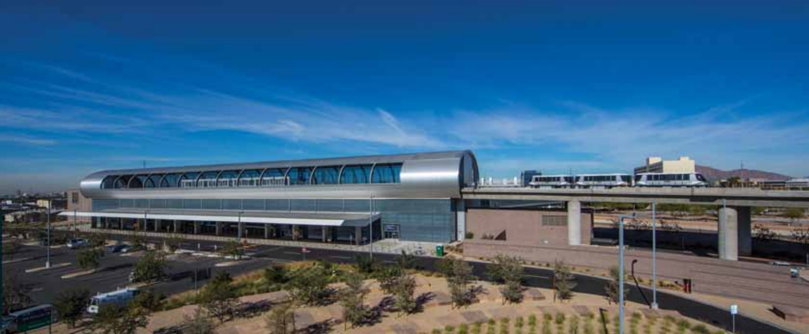
44 th Street Station. Courtesy of Bob Perzel.
