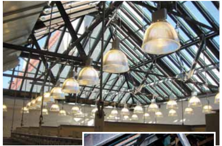
Figure 4: Assembly Staircase attic before and after installation of new skylight, laylight, and staircase lighting. Before photo courtesy of Laurie Donald, Bernstein Associates Photographers, for OGS.
