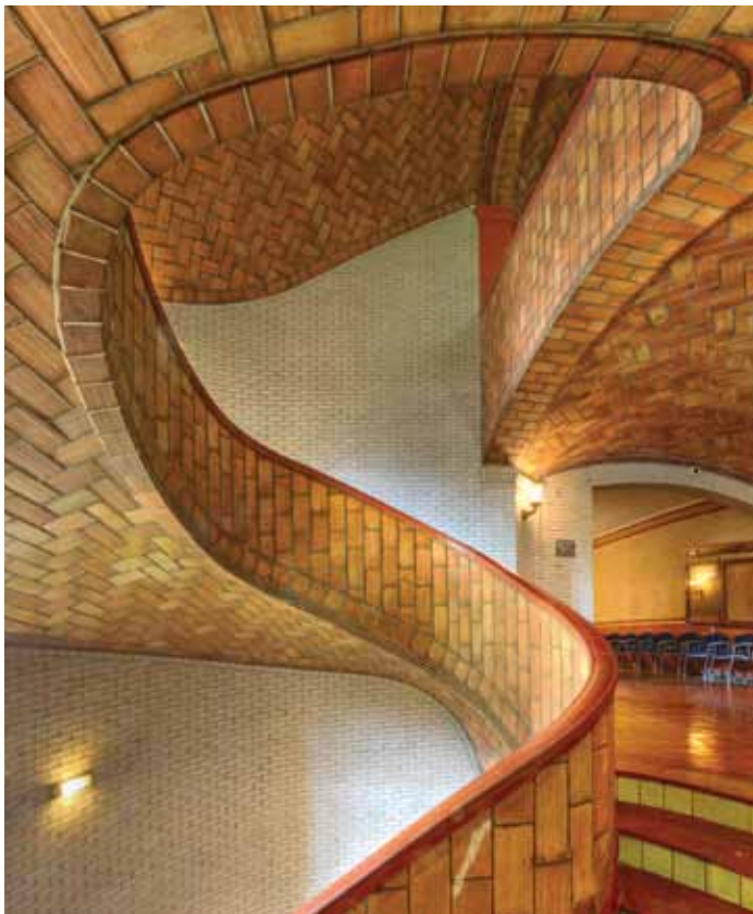
Figure 5. Tile vaulted staircase of Baker Hall, Carnegie Mellon University, Pittsburgh, 1914. Courtesy of Michael Freeman.
