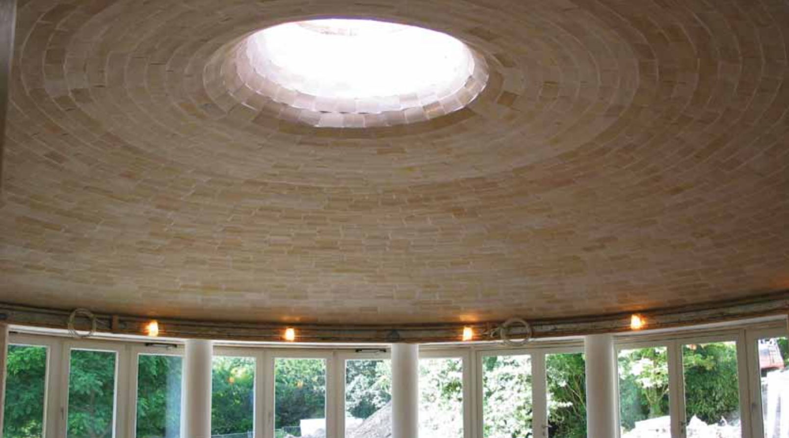
Figure 7. Structural tile dome, Pines Calyx, St. Margaret's Bay, England (2005).
