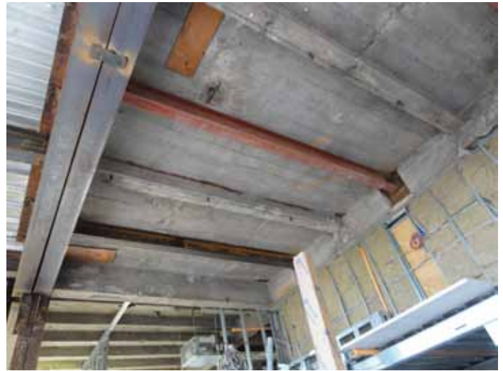
Figure 4: Existing beam and slab strengthening.
