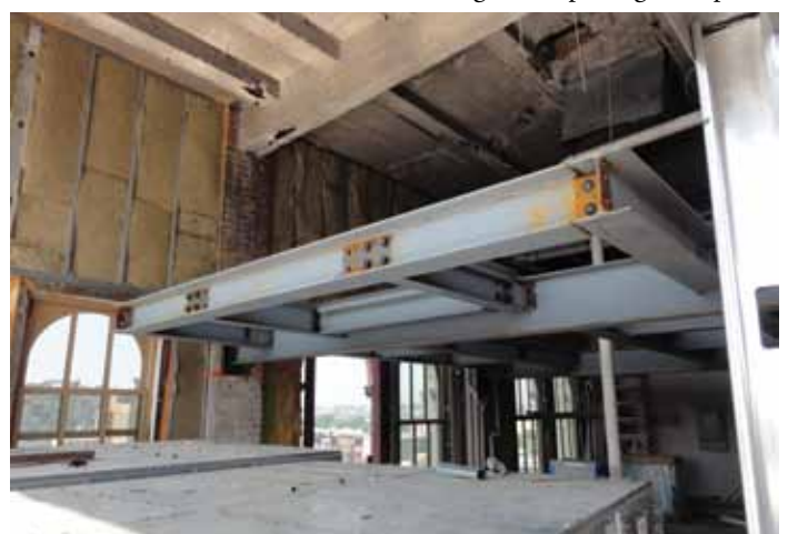
Figure 5: New 12 th floor interior dunnage frame.
