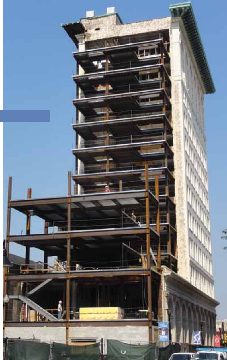
Figure 1: Partially erected stair and addition framing.
