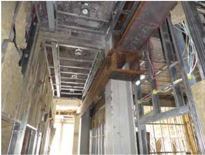
Figure 3: New transfer girder connection at existing column.
