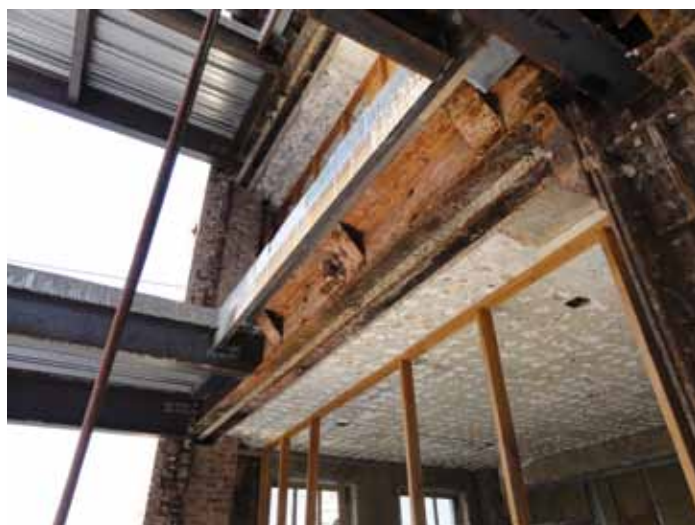
Figure 2: New tie-in conditions at existing spandrels.
