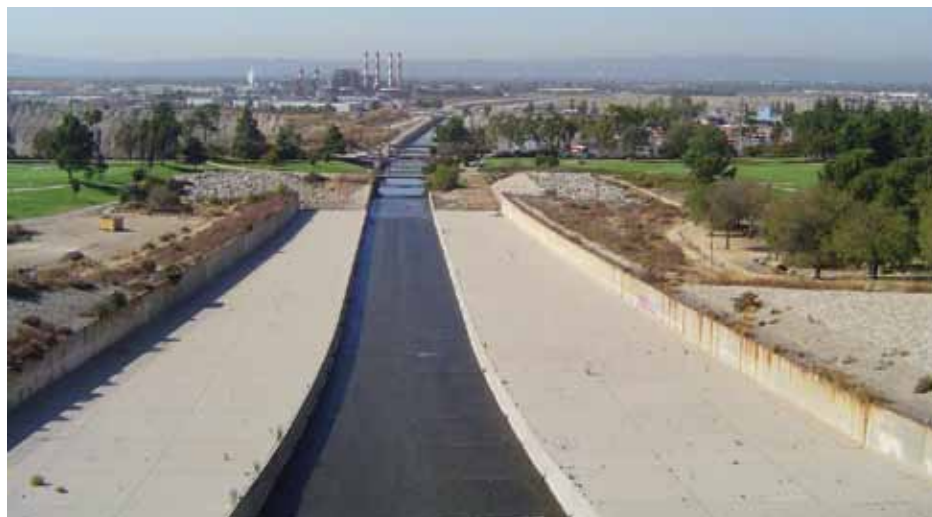
Three bridges crossing the Tujunga Channel: golf cart bridge, crossed arches pipe bridge, and rubber dam maintenance bridge. Red and white stacks in background are at Valley Generating Station, site of the recycled water Hansen Tank and Pumping Station.
