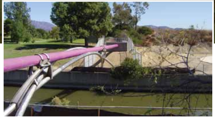
View of the completed crossed arches pipe bridge.
