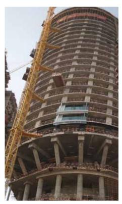
installed as an attractive structural solution. The hangers are supported by a deep Post Tension beam at the Podium Roof where clear height was not a major issue.
