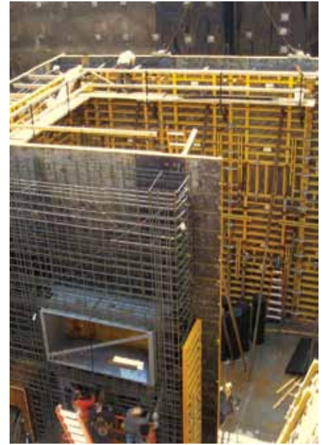
Preparations for the 40-foot tall concrete vault pour.
