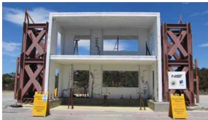
Research was part of the process used to develop Limit Design. This full scale, 2-story masonry specimen with irregular openings was tested on the shake table at UC San Diego as part of a NEES/NIST funded project. Courtesy of Richard Klingner.
