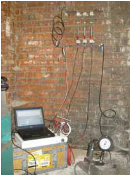
Figure 3: Masonry deformability test by the Flatjack method to estimate masonry compressive strength and elastic modulus. Both Flatjacks are pressurized while monitoring surface strain to generate an in-place stress-strain curve.
