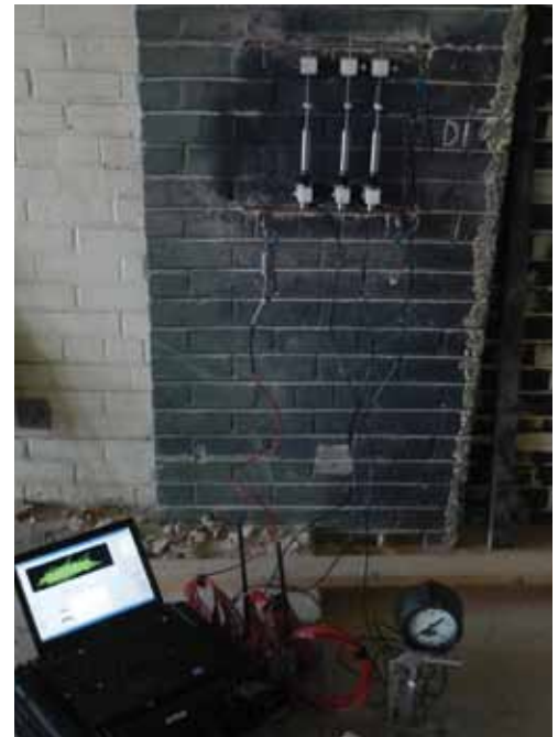
Figure 2: Flatjack deformability testing to measure masonry elastic modulus and estimate compressive strength.
