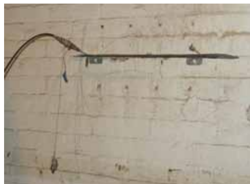
Figure 1: Single flatjack test used to determine masonry in situ stress.
