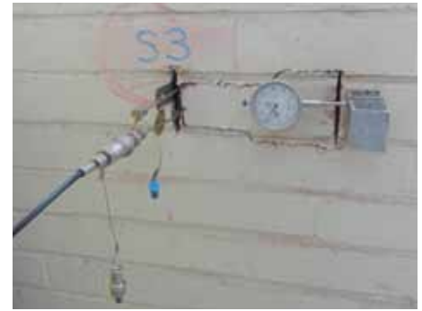
Figure 4: Masonry shear strength testing using a specially-sized flatjack.
