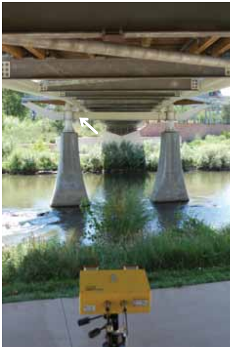
Figure 6: IBIS set-up beneath cable-stayed bridge.
