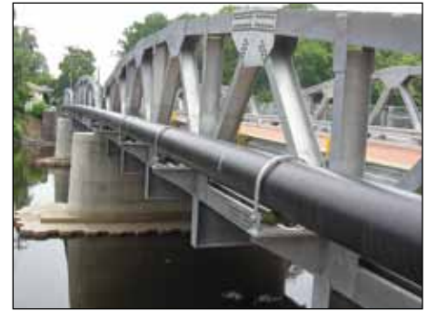
Bergen County, New Jersey Hot-dip Galvanized Short-Span Bridge.
