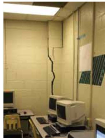
Figure 5: Masonry damage in Louisa County. Non-structural components damage from Louisa County High School (GEER Photos by R. Green, EERI Clearinghouse, eeri.org ).
