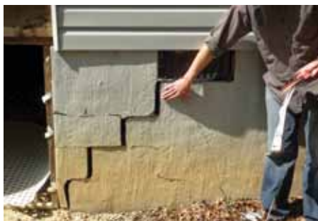
Figure 5: Masonry damage in Louisa County. Non-structural components damage from Louisa County High School (GEER Photos by R. Green, EERI Clearinghouse, eeri.org ).
