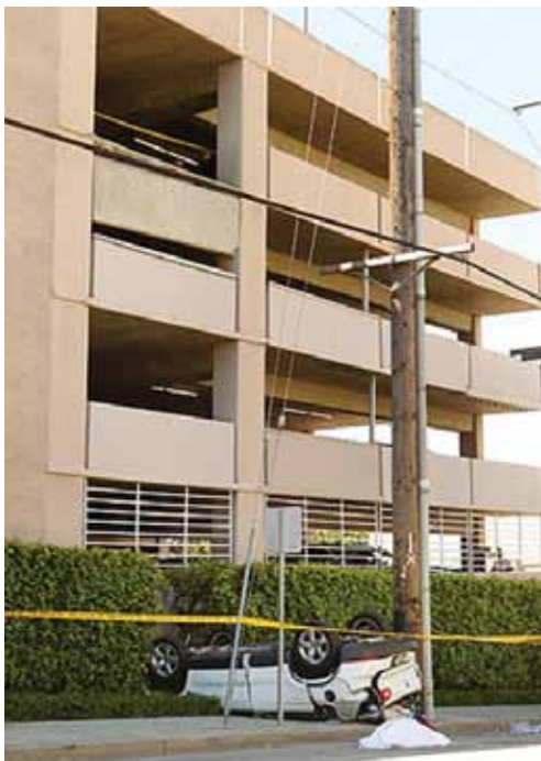
Figure 1. Barrier wall failure and car plunges down.
