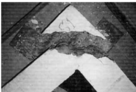
Figure 3. Brittle mode failure of slab-wall type joint under opening moment.
