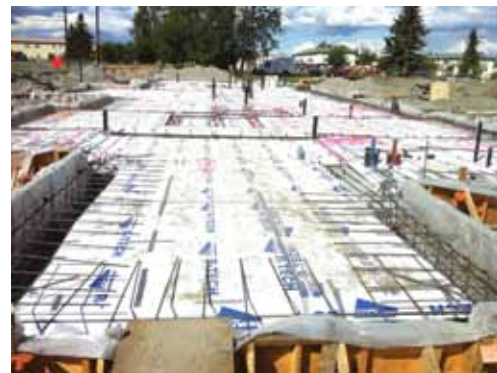
EPS insulation in an under-slab application. Courtesy of Insulfoam.
