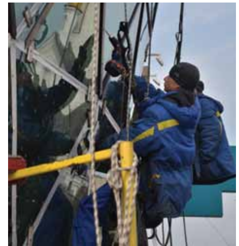
Figure 4: Installing elements by working with climbing equipment.
