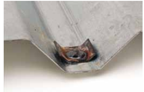
Arc spot weld with weld washer.
