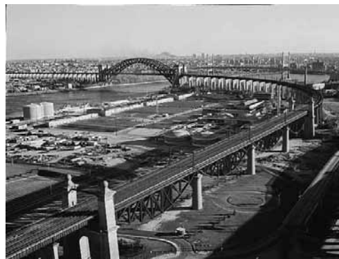
Recent overview of the project looking south, showing the flagship Hell Gate Bridge and the 4-span Little Hell Gate inverted bowstring arches in the foreground. Towers probably by Henry Hornbostel, Architect. Courtesy of www.loc.gov . HAER, NY-121-16. G. Weinstein, Photographer. 1996.
