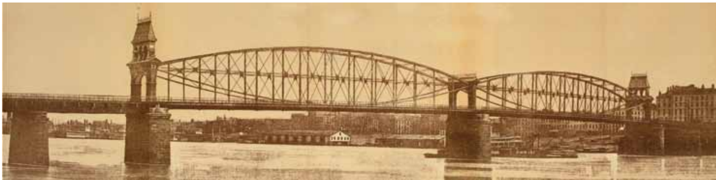
Lindenthal 1881 office illustration: "View of the Two Channel Spans", showing the massive one-bay-wide, original steel-supported and embellished with iron portals, under a three-bay-wide arcade supporting a mansard roof. Transactions of the ASCE , Vol. XII, Plate XXII. Sept. 1883.
