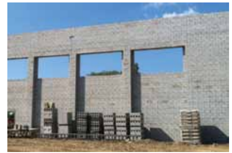
Figure 4. Masonry walls under construction utilizing internal bracing. Courtesy of Koch Masonry, Dexter, Michigan and IMI – Internal Bracing Guide.
