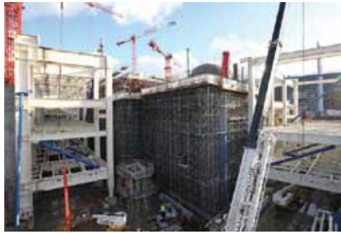
Figure 1: Conventional cast-in-place turbine generator deck (1,600 MW).
