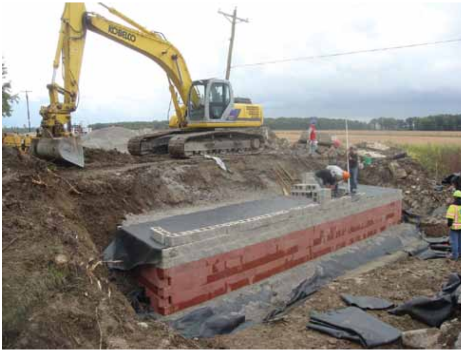
GRS-IBS technology, which uses layers of compacted granular fill and fabric sheets of geotextile reinforcement to provide bridge support, is part of FHWA's Every Day Counts initiative to accelerate project delivery.
