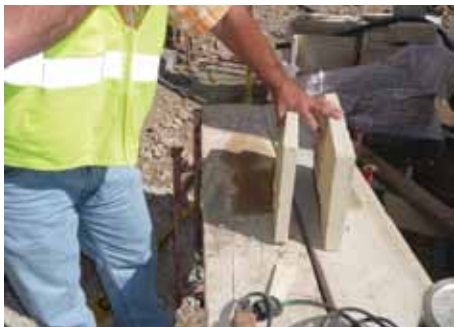
Substantial differences in thicknesses are found in these two natural stone units, even though they are from the same batch.
