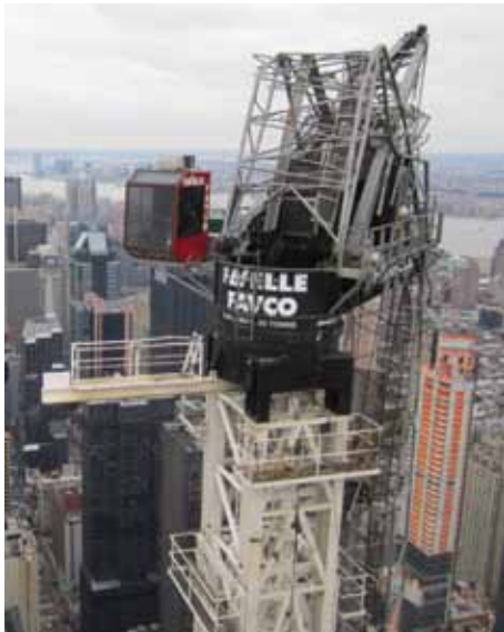
Figure 6: A tower crane boom flipped backwards during Hurricane Sandy, dangling above the streets of Manhattan.
