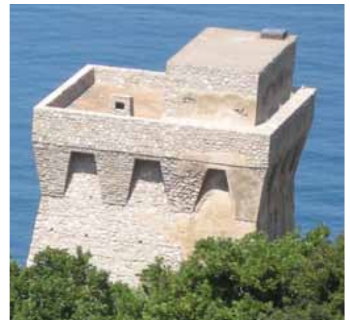
Medieval tower with masonry corbels.
