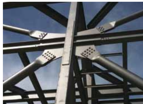
10.750- and 8.625-inch diameter braces equipped with Cast ConneX High-Strength Connectors framing into a “butterfly” gusset plate connection at the beam-column intersection.
