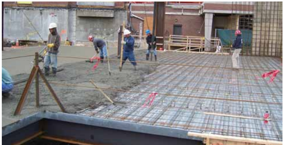
Figure 2: Placing lightweight concrete on composite metal floor deck. The metal floor deck allows the concrete to dry only through its top surface.
