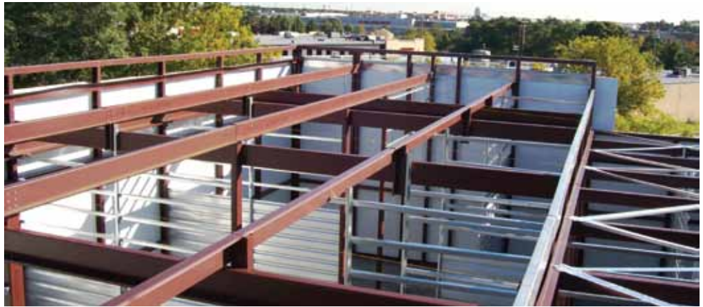
Figure 1: Roof and wall framing.
