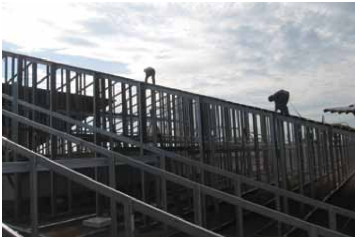
Figure 3: Cold-formed steel for roof retrofit at MacDill AFB in Tampa, FL.
