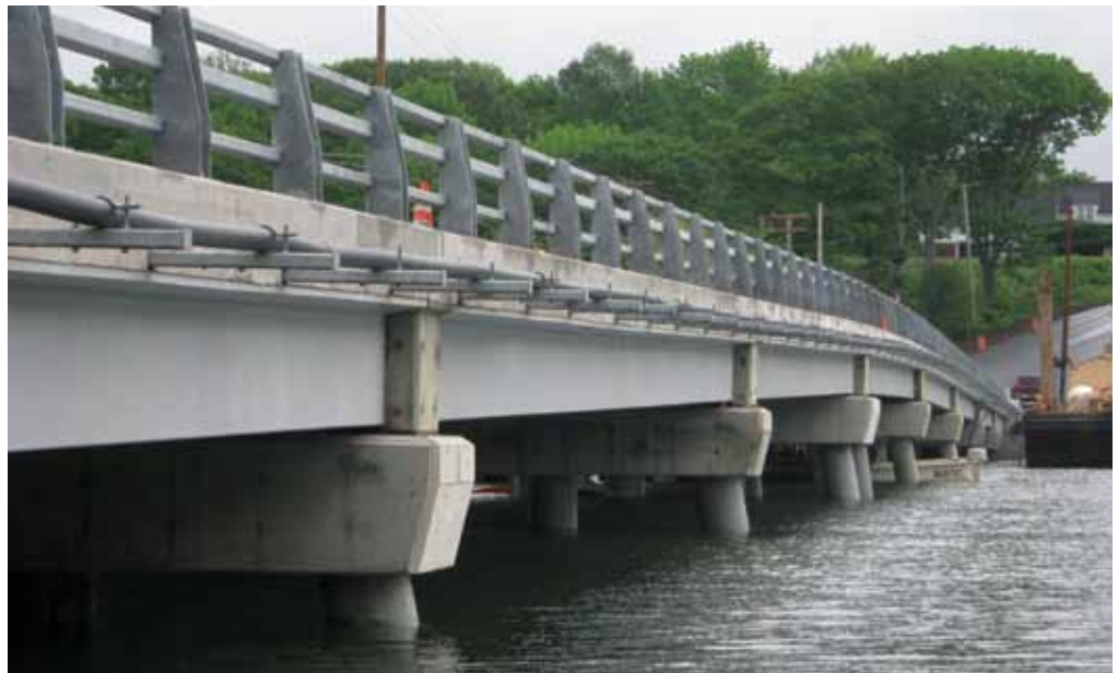
Knickerbocker Bridge in Boothbay, Maine.
