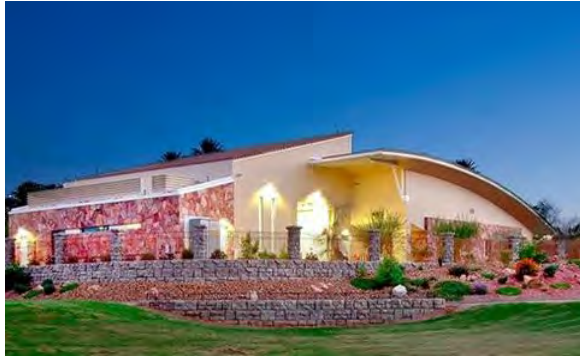
Fire Station, Las Vegas, NV
